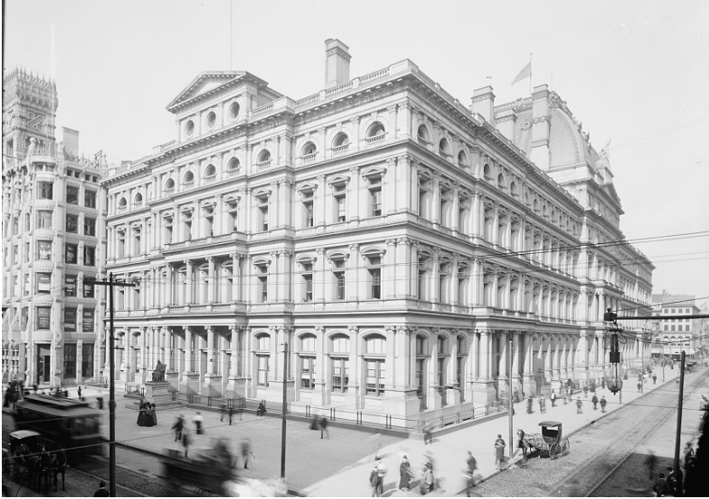
U.S. Post Office and Court House, Philadelphia, Pennsylvania. Source: Library of Congress, Prints & Photographs Division, repro. no. LCDIGdet4a08430 (ca. 1900).
